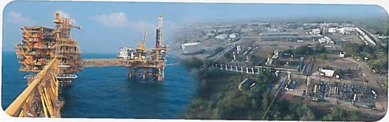
Offshore Platform, HPHT Asset
